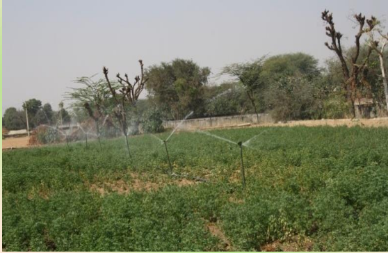
Sprinkler system installed at SKNCOA, Jobner
