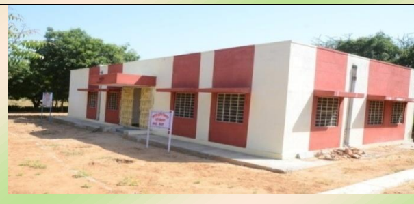
Hatchery building constructed under Backyard Poultry Project
