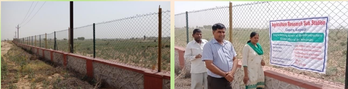
Construction of boundary wall to protect ARSS farm.
