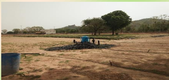
Micro irrigation, solar water lifting system with generator and inverter
