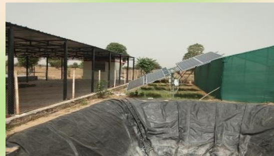
Construction of water harvesting structure
