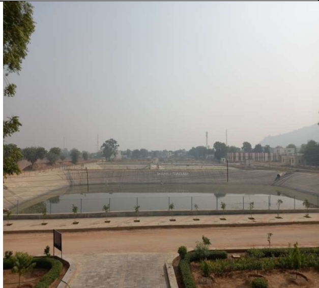
Rain water Harvesting Structure
